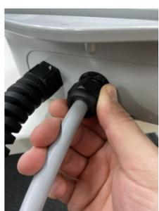
9. Connect the supply cable in accordance with the local wiring regulations. Strip back 10mm of insulation from the wires on the mains cable.
