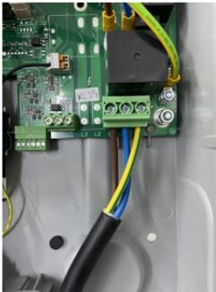
10. Connect any relevant CTs into the termination blocks provided. **The CT Golden Rules must be followed for the zappi to work correctly**
